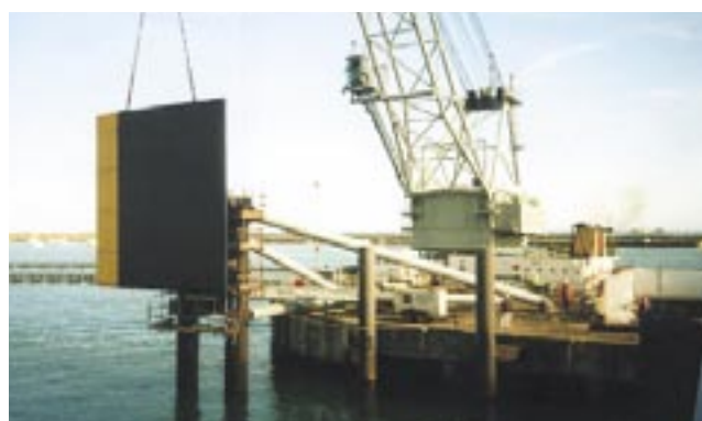
▲ During installation of Dunlaoghaire HSS Berth (IRELAND)
