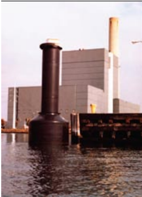
▲ Corner Protection, Tanker Dock, New Haven, Connecticut, USA
