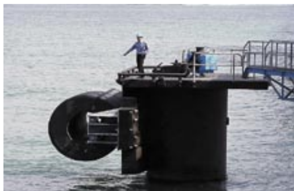
▲ Power Station Coal Berth
