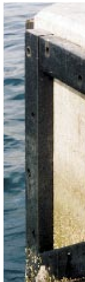
▲ Corner protection (DUBAI)
